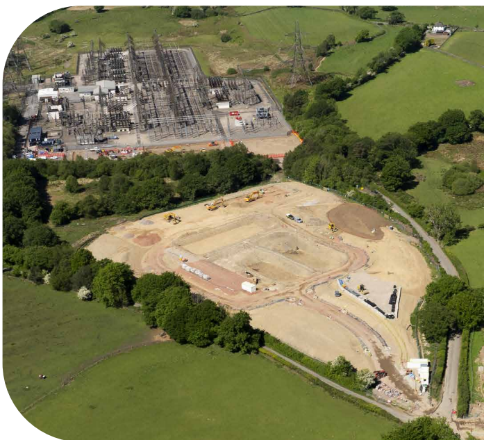
Figure 18: Cilfynydd construction site
