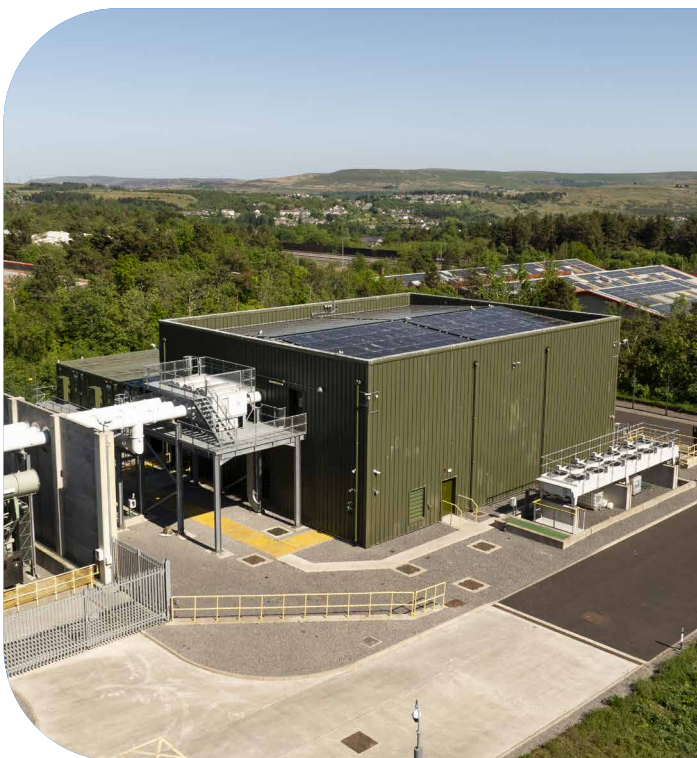
Figure 17: Rassau synchronous condenser site shown for illustrative purposes
